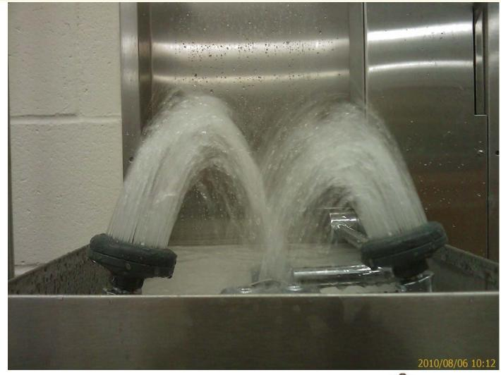
This eyewash is deficient. Nozzle flow is low with the flows barely making it to the center of the eyewash mount.
