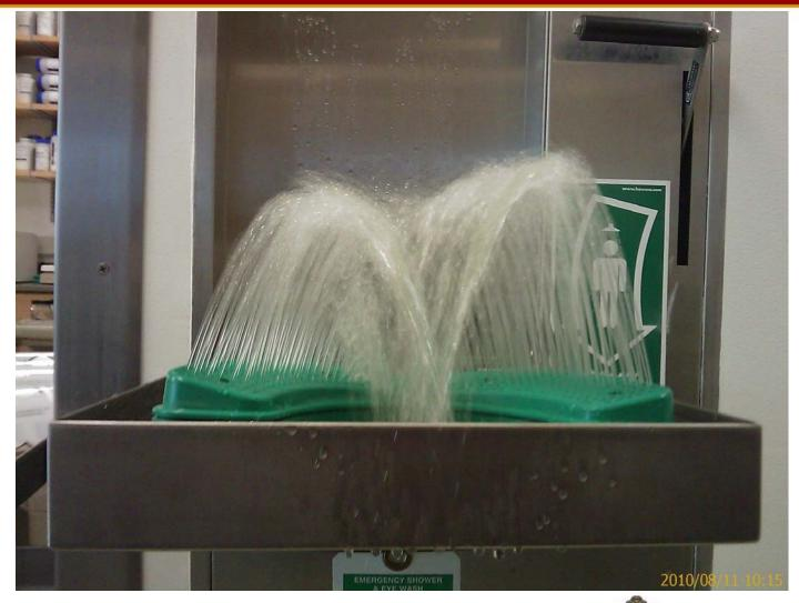
This is a good example of the face wash kind of safety eyewash. Flow is good and near uniform with a height of six inches or greater.
